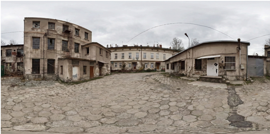
The current state of the courtyard
